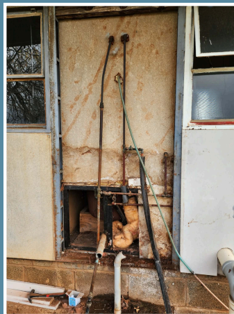
Opened wall view of old plumbing
