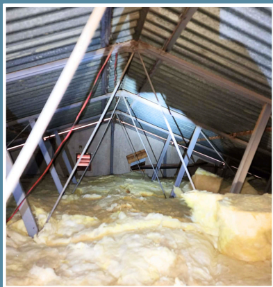
Added insulation in ceiling
