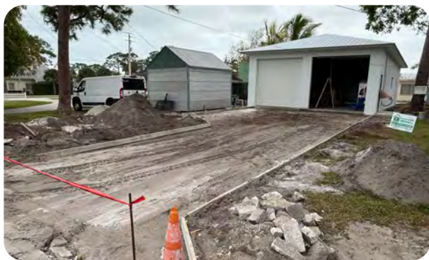
New GPM and FEA storage building
